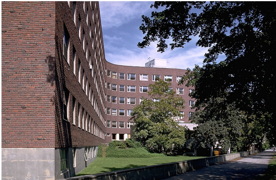
Figure 17: Alvar Aalto, Baker House, 1947, renovated Perry Dean Rogers, 2002
